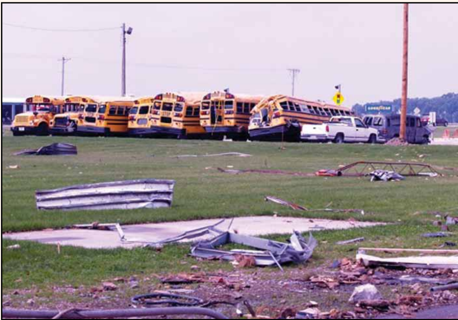
Buses at the Lake Local (Wood) High School following the June 2010 tornado.
